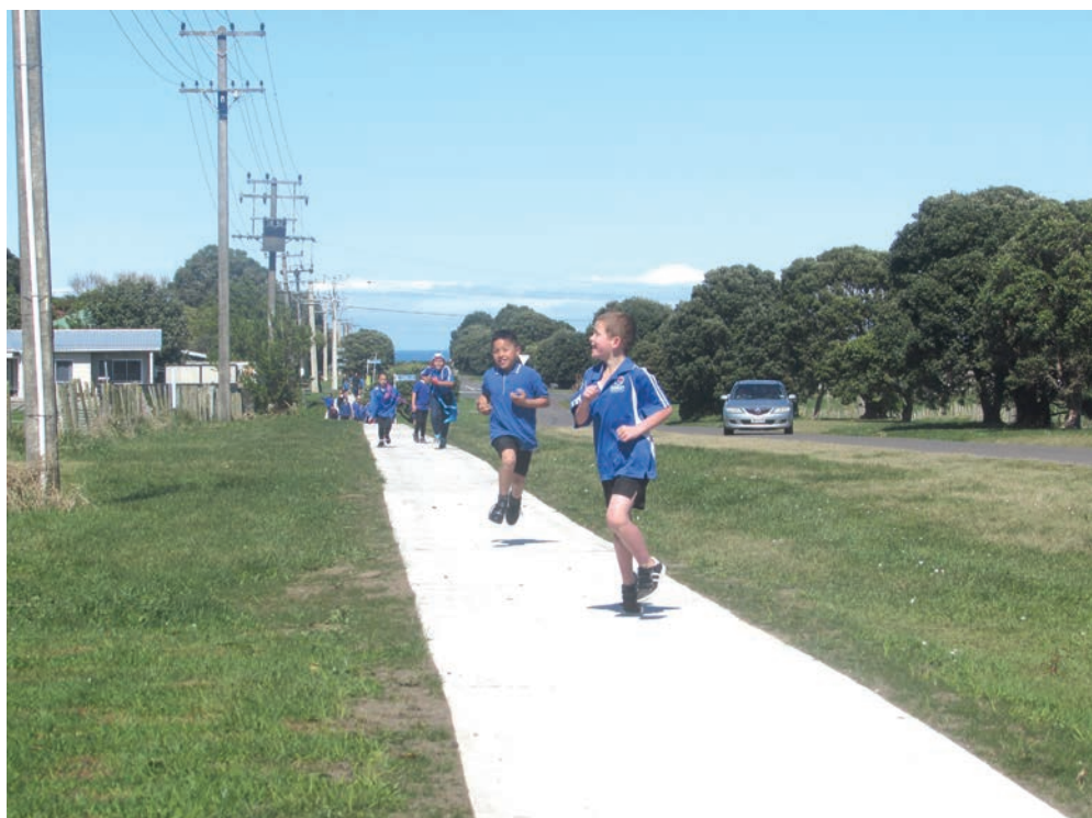
Look at this. Manaia Primary School pupils take to the new footpaths.
